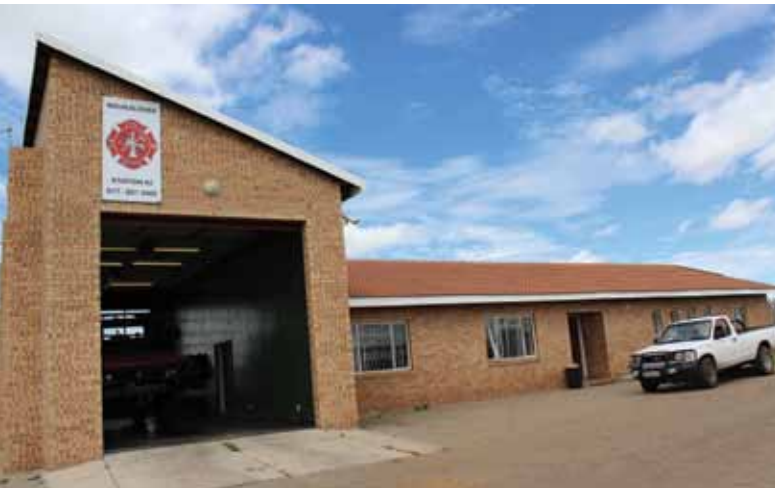
Msukaligwa Fire Station #2 in Breyten, Mpumalanga
