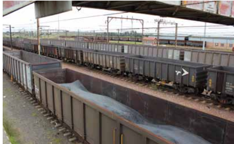
The Transnet railway link between Msukaligwa and Richards Bay in one of the major fire risks in the municipality
